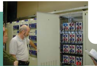
Inspection of energy installations (Champagne-Ardenne – eastern France)
