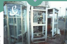
Plastics, rubber, metals and other materials are the principal waste products generated by France Telecom. Storage of retired telegraph poles prior to recycling.
